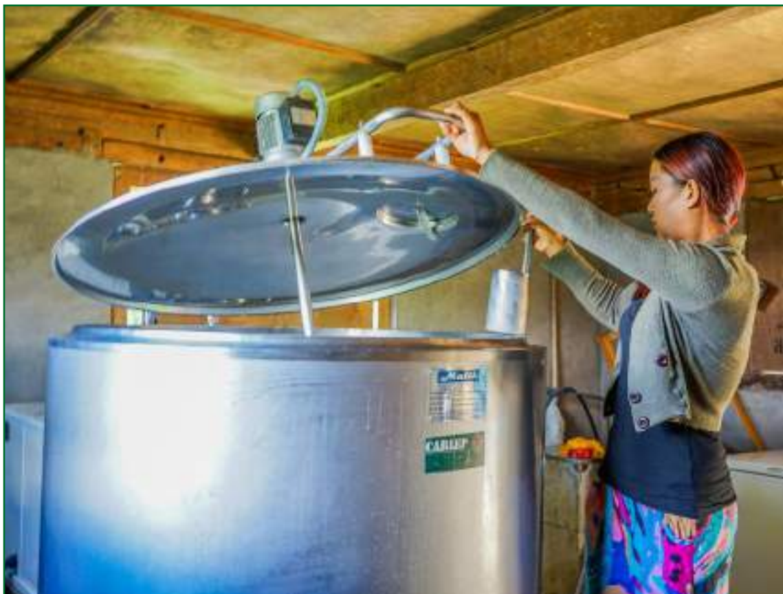
Milk Chiller installed at Khabtey MCC with supports from CARLEP
