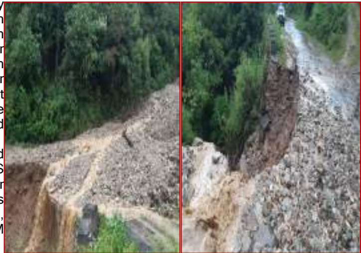
Figure 22. Flash flood of September, 2021 damaging approach road
