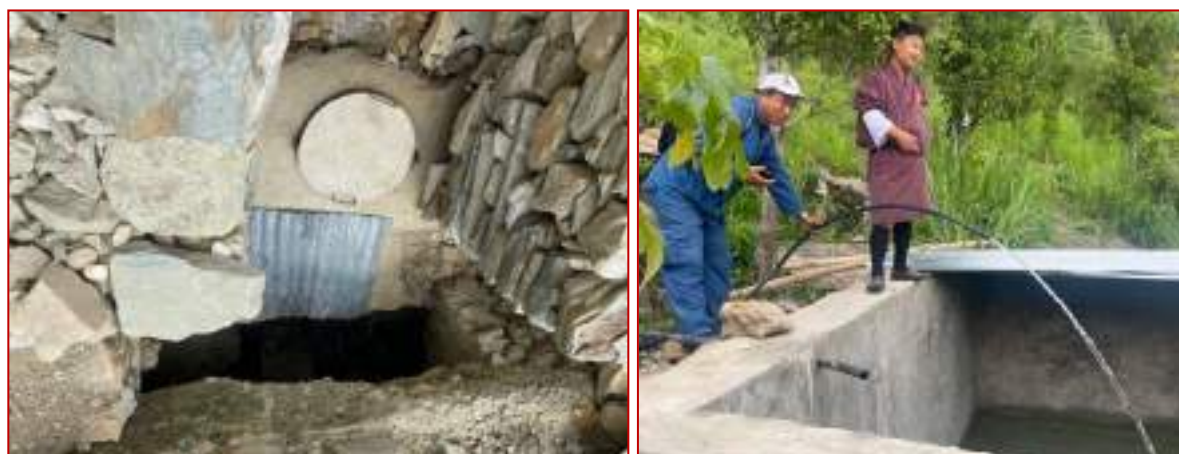
Figure 33. New source collection tank (left) and service tank (right)
