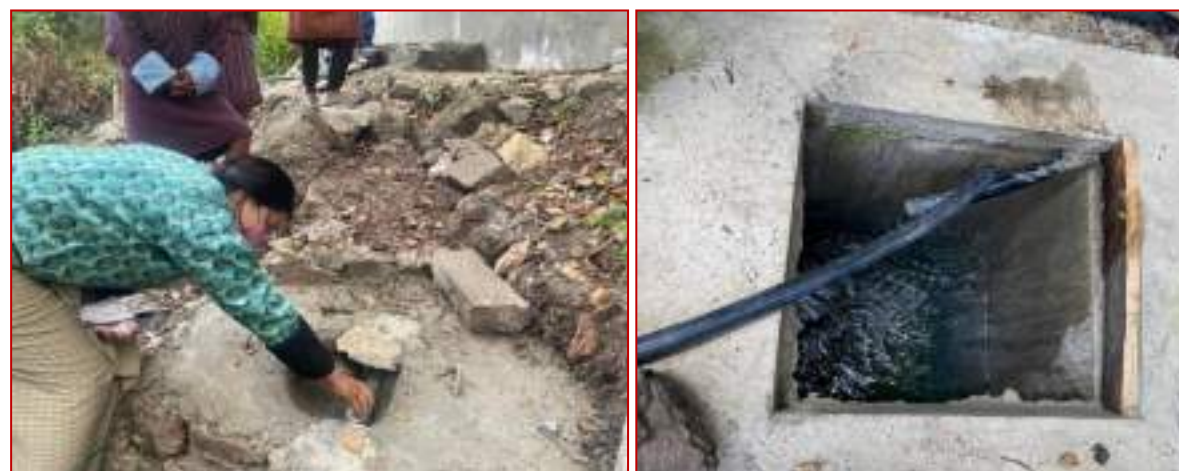
Figure 34. Gate valve for mainline (left) and reservoir tank (right)
