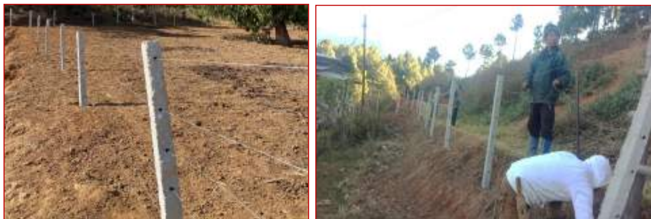
Figure 36. EF using concrete poles installed
